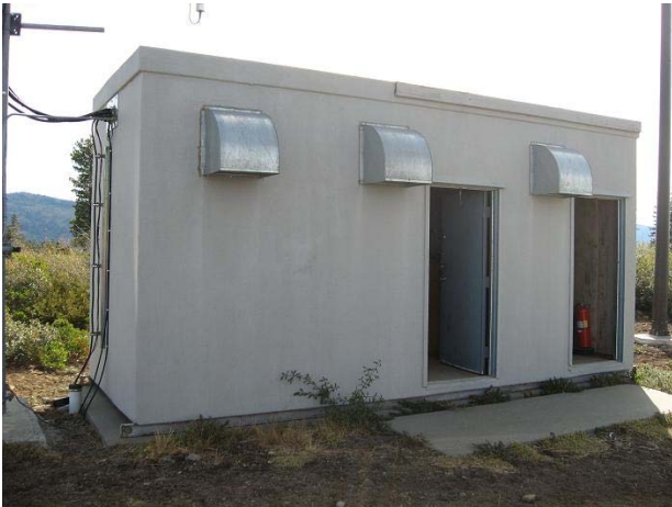
A new pre-fabricated radio vault with superior security, stability and life expectancy.
