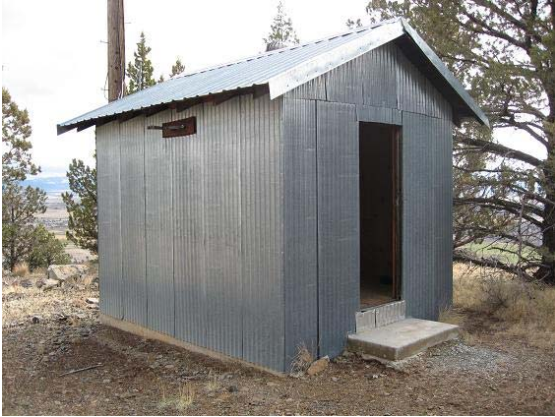
The existing radio vault located at Barnes Grade.
